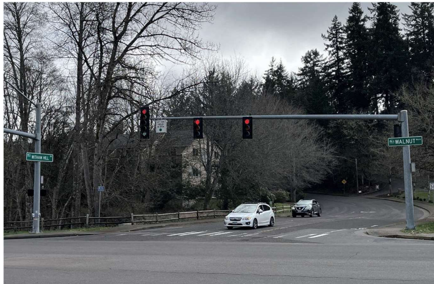
FIGURE 3: LEFT-TURN SIGNAL HEAD WITH RED BALL AND GREEN ARROW
