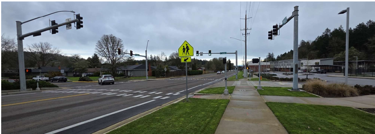
FIGURE 16. NW ASPEN STREET INTERSECTION WITH BESSIE COLEMAN SCHOOL ENTRANCE
