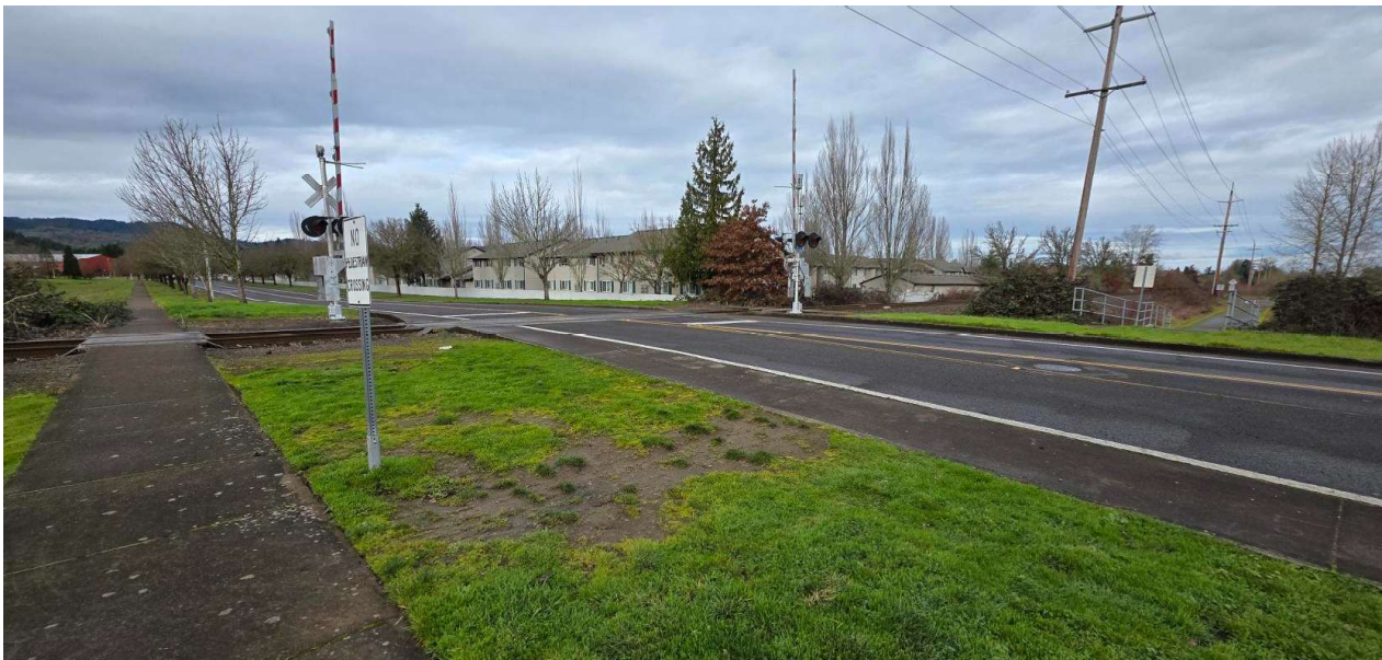
FIGURE 12. EXISTING RAILROAD CROSSING WITH SHARED USE PATH AND NO CROSSING SIGNAGE
