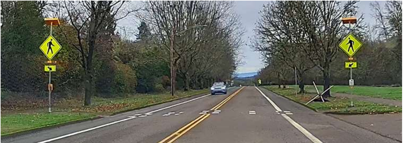
FIGURE 17. RRFB ENHANCED CROSSING AT MLK JR. PARK
