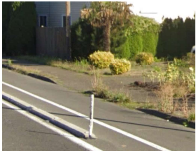
FIGURE 7: EXAMPLE OF CONCRETE ISLANDS (IMAGE SOURCE: GOOGLE STREETVIEW)
